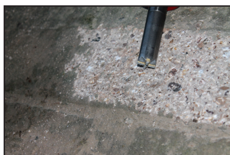
ROUGHENING CONCRETE
