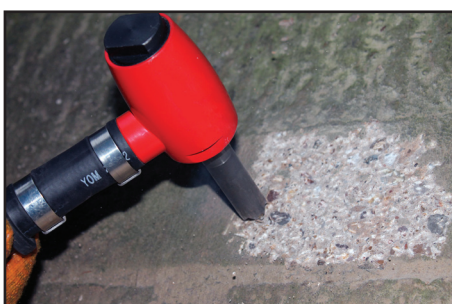
REDUCING LEVELS ON CONCRETE
